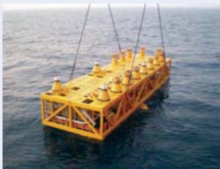
The deepwater pipeline end manifold (DWPLEM) being installed.
