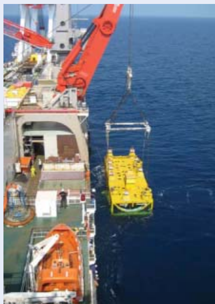
Allseas' Audacia installing a PLEM
